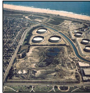
Ascon Landfill Site Huntington Beach, California
